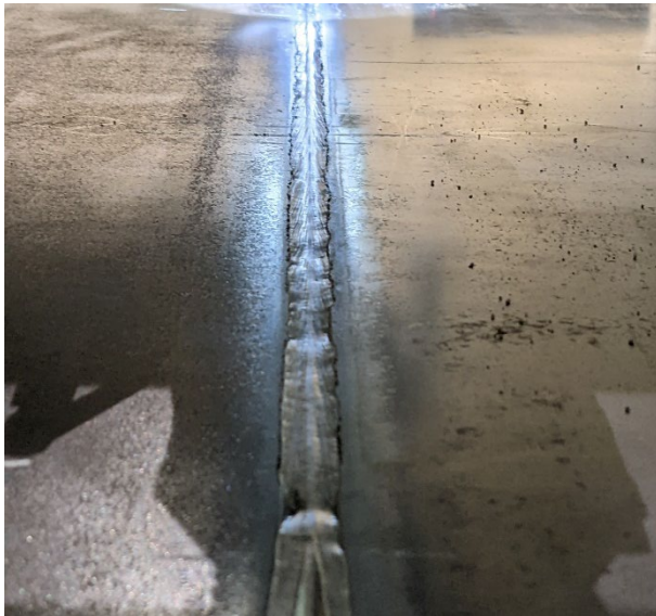
Figure 37. Visually Inspect Cleaned Welds (Left) First Pass (Right) Second Pass
