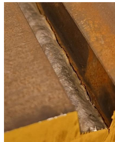
Figure 12: Welding pass showing cracking in the base material – see the crack line running along right edge of filler material
