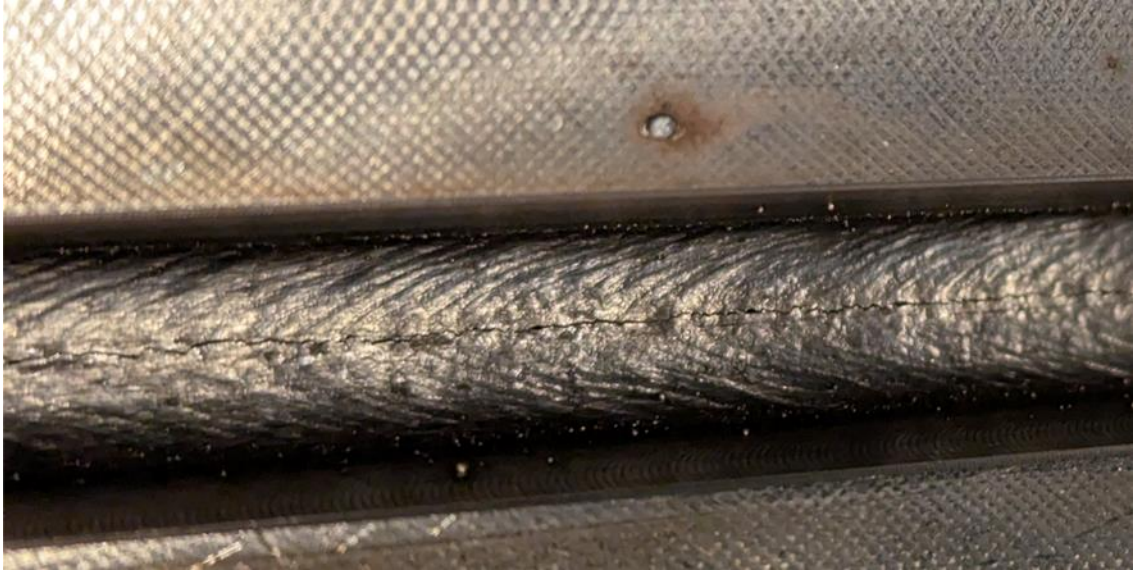
Figure 69. Centre line cracking seen in the filler material
