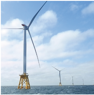
6 MW Block Island Turbines Rhode Island State Waters
