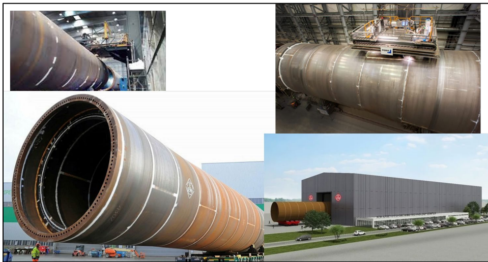
Figure 27 Spar Fabrication uses Proven Manufacturing Techniques for Monopiles (Source: EEW Group)
