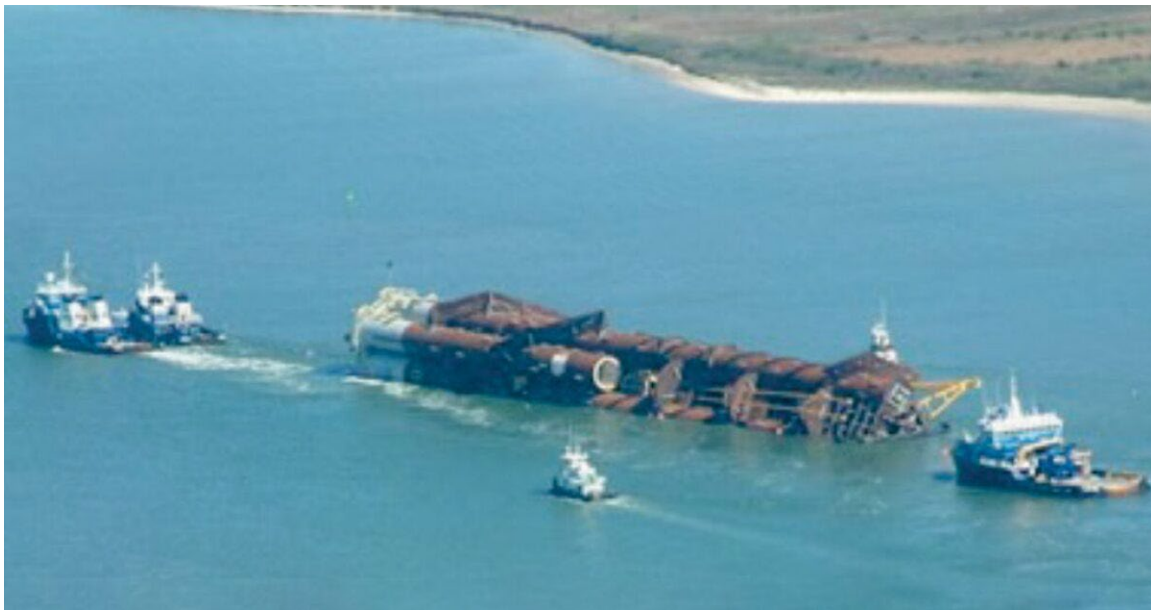
Figure 37 Red Hawk Cell Spar Being Towed after Loadout 6
