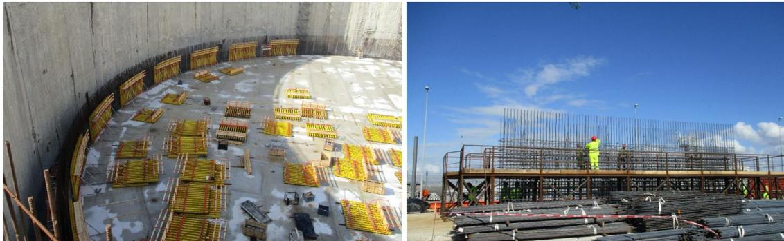
**Figure 68. Preassembled reinforcement**
