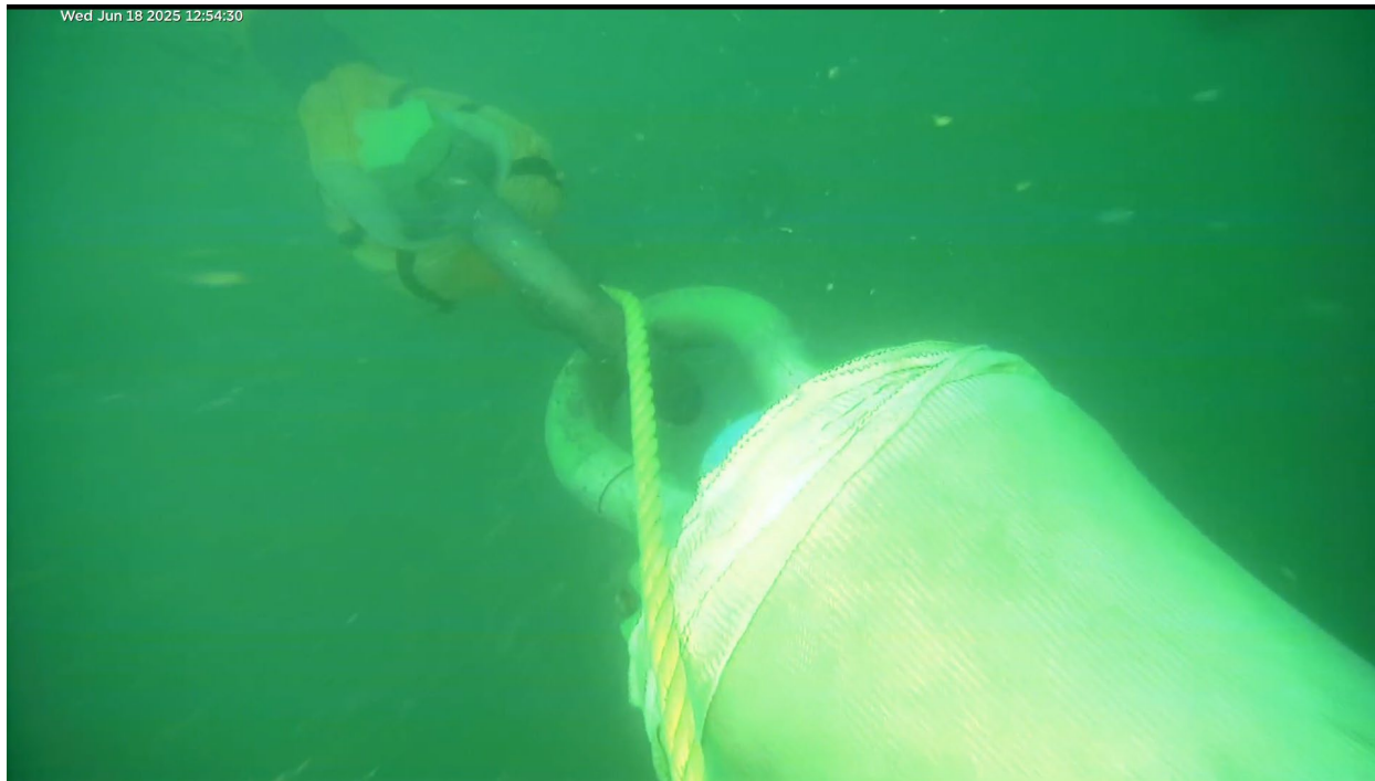
4m IMS end flange (without air connection) with 2" and 2" wide jaw shackles connected to 2.5" HMPE thimble.
