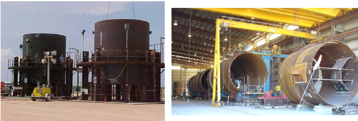
Figure 19. Suction pile manufacturing and assembly of cans and supporting jigs.
