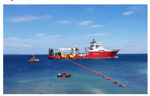
Figure 6-12: Landfall Pull-in with cable floated from the CLV towards shore.
